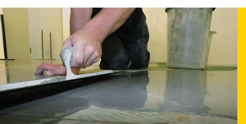
F. Ball floor smoothing compounds provide bespoke solutions for a wide range of conditions to ensure an ultra-smooth, durable finish ready for the installation of the final floorcovering.
